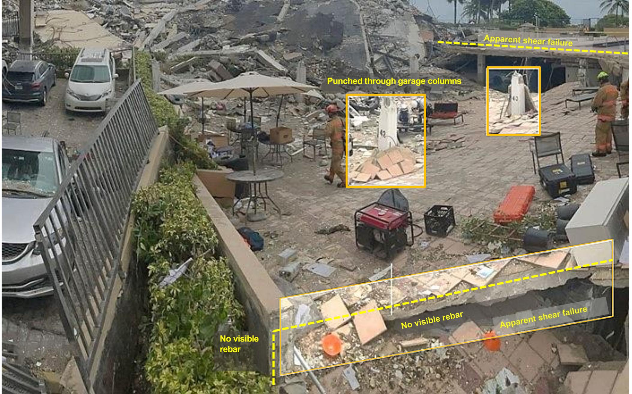
**(B)** Parking deck over garage, collapsed into garage below
