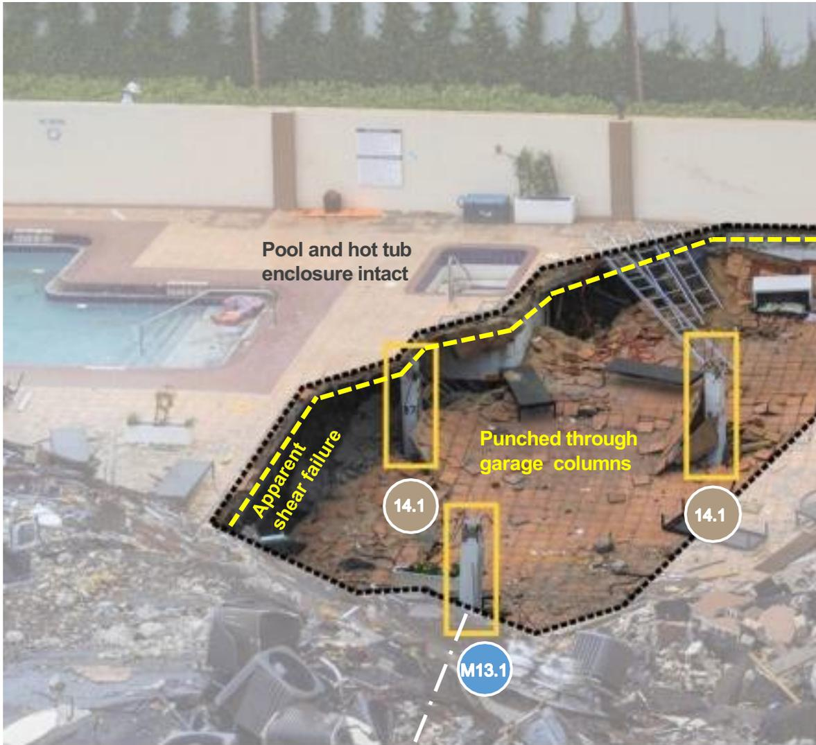
**(A)** Pool deck with punch through of columns down to garage
